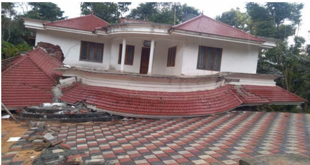
Photo 1: building collapsed due to rotational landslides at Mavadi Idukki district
