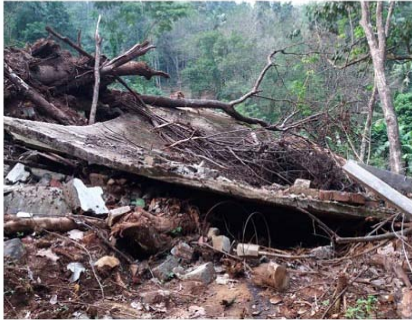
Figure 7. Ferocious landslide left only the concrete roof of the building. Building strong houses with column and beam would be better than building houses with load bearing wall system. First question is whether it is safe to construct a house in landslide prone areas!
