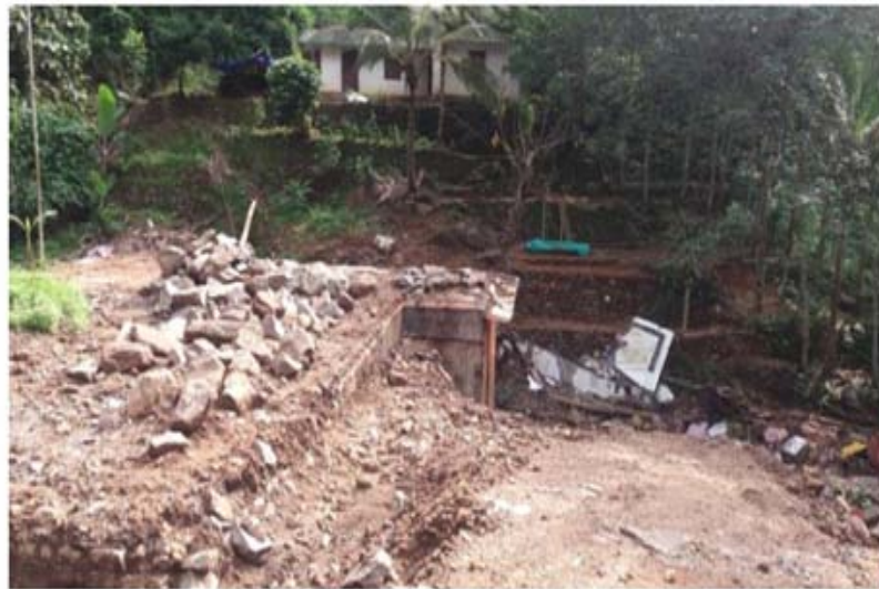
Figure 2. Though this house which fully got destructed in landslide was situated in a comparatively gentle slope, this house was impacted due to a landslide which occurred in the opposite hill. The debris from the landslide crossed the valley and destructed the house.
